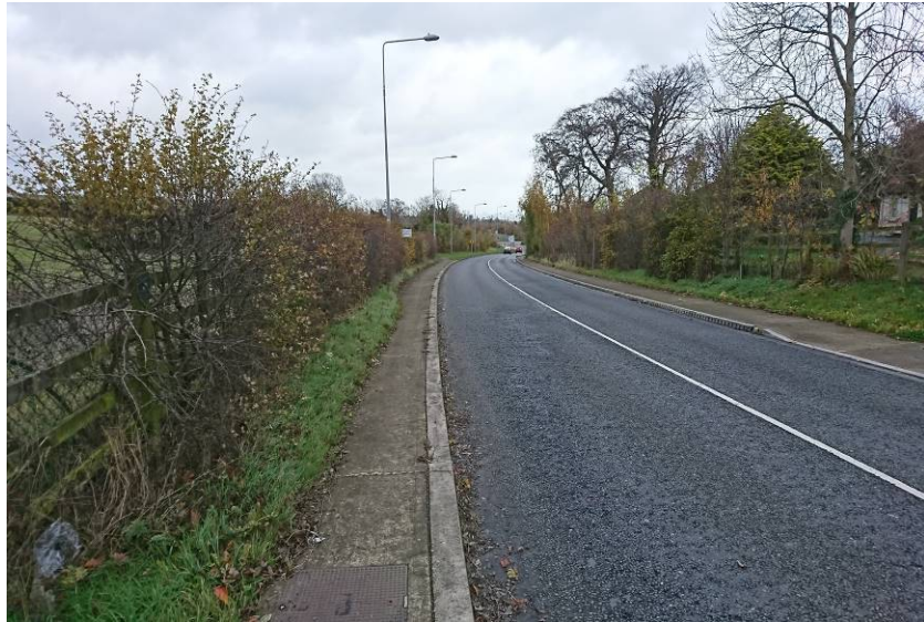
Plate 1 R751, facing north
